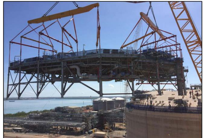
**Propane Platform Lift – 516 tonnes on the Crane Hook.**
