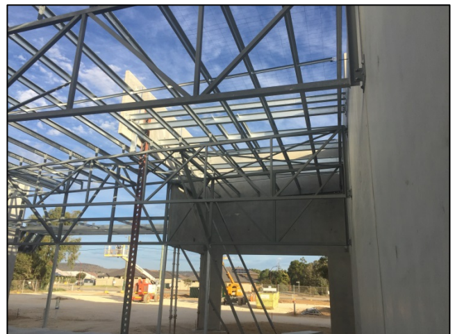
Entrance Structure (March 2016)
